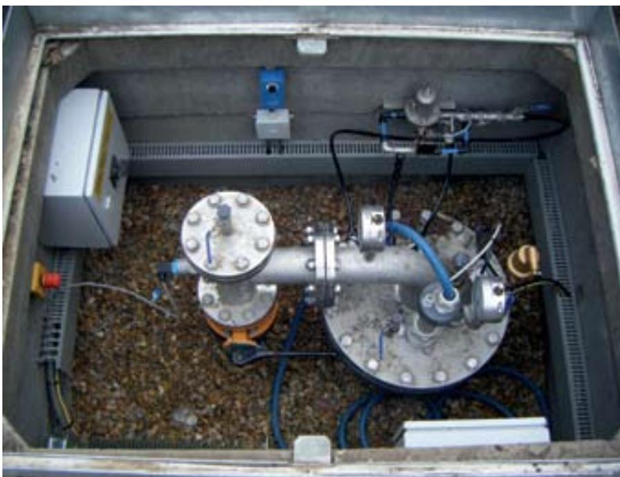
Top: Plant room showing the prefabricated, skid-mounted unit containing the plate heat exchangers and control valves
