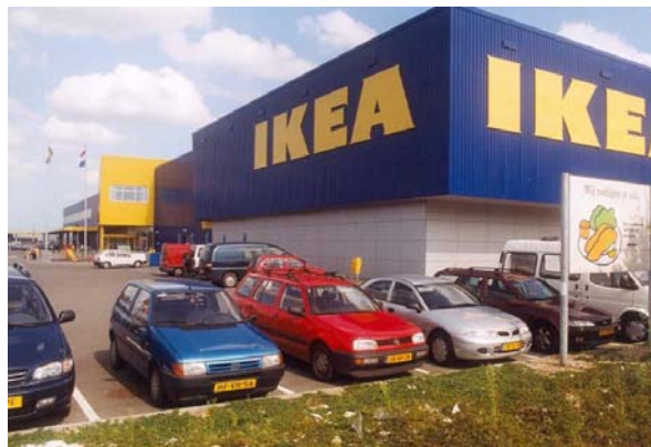
Figure 5. IKEA store, Duiven. ATES cooling (600 kWt (170 Tons)) and low temperature heating according to system concept 2.
