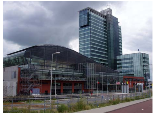
Figure 6. Mixed use project, Amsterdam. Heat pump system and ATES cooling ( 4,500 kWt (1,300 Tons)) according to system concept 3.
