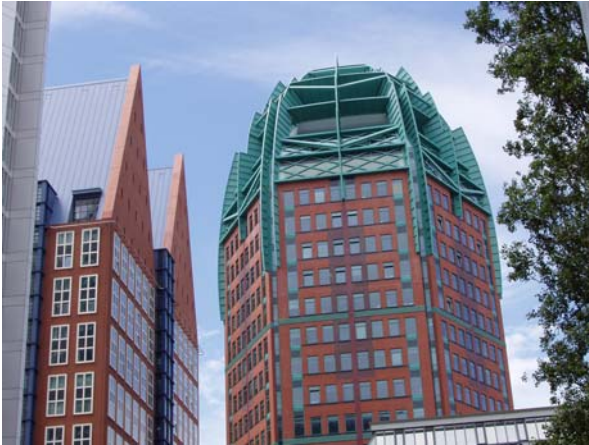
Figure 4. “De Resident” offices, the Hague. ATES cooling ( 2,500 kWt (710 Tons)) according to system concept 1.
